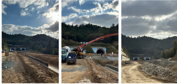
Figure 3. A view of the Construction Site
